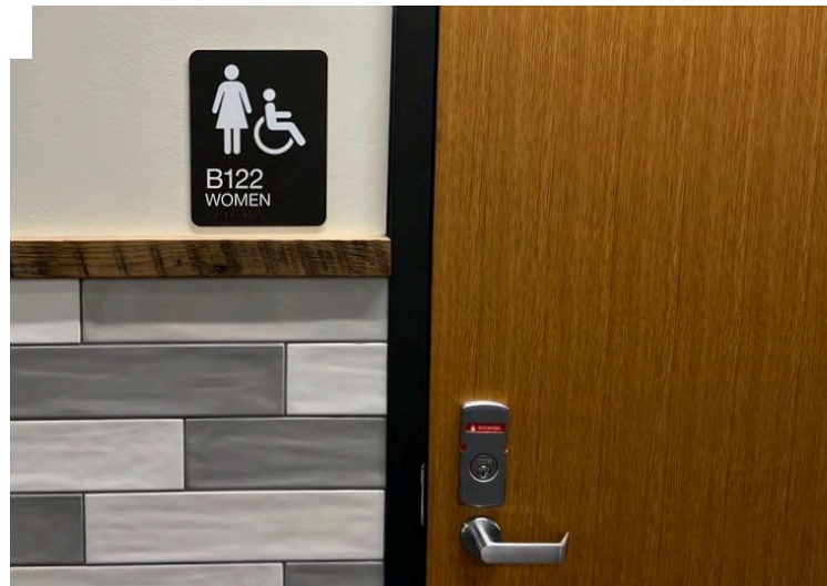
9"x7" acrylic ADA sign with dimensional letters, pictogram and braille.
