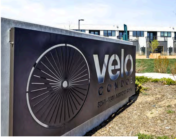
Illuminated 4'x8' precast concrete monument sign with anodized black aluminum face and cutout copy
