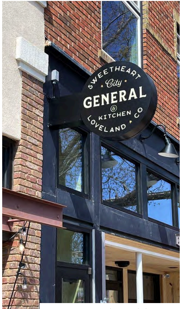
4' projecting, round painted aluminum cabinet, illuminated with routed and backed copy.
