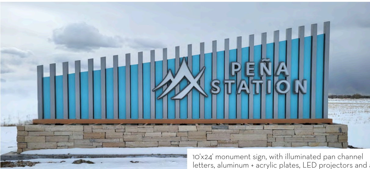
Illuminated, aluminum monument sign with vinyl overlay and decorative seams
